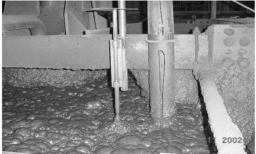
Figure 13: New Level Control system and old tube type system alongside
